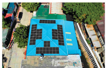
21.45kW Solar Grid-Tied System Quirino
