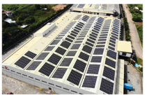
1.5MW Solar Grid-Tied System Silang, Cavite
