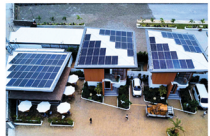
99kW Solar Grid-Tied System Botolan, Zambales
