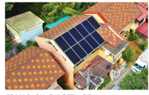
5kW Solar Grid-Tied System Quezon City
