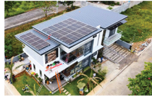
10kW Solar Grid-Tied System Waterwood, Baliuag, Bulacan
