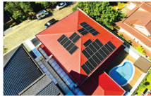
15kW Solar Grid-Tied System Corinthian Gardens, Quezon City
