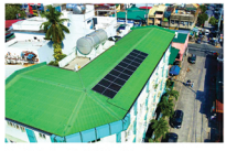
5kW Solar Grid-Tied System Laloma, Quezon City
